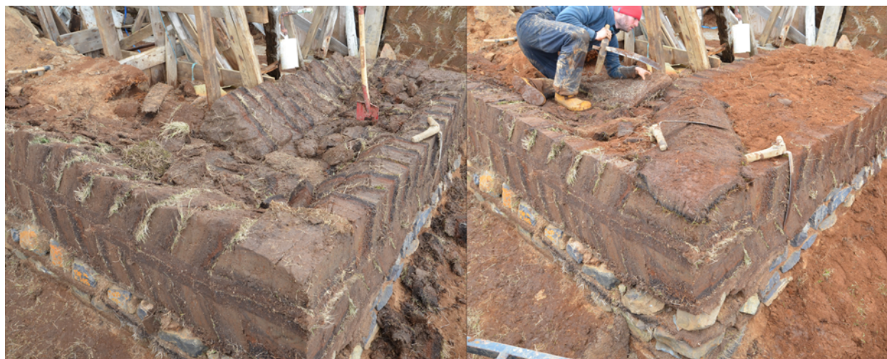
Figure 4.10 Icelandic turf wall construction: herring-bone facades of klambra or 'clamped block', and alternate courses of strengur , with an earthen/turf core on a dwarf foundation wall (D. Strachan: 2013).
